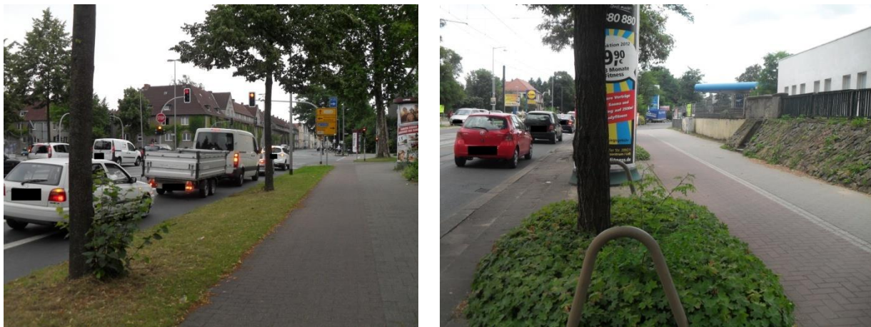
Figure A.8. Examples of separated cycle lanes with potential line of sight obstruction in Germany. Source (Schreck & Seiniger, 2014)
