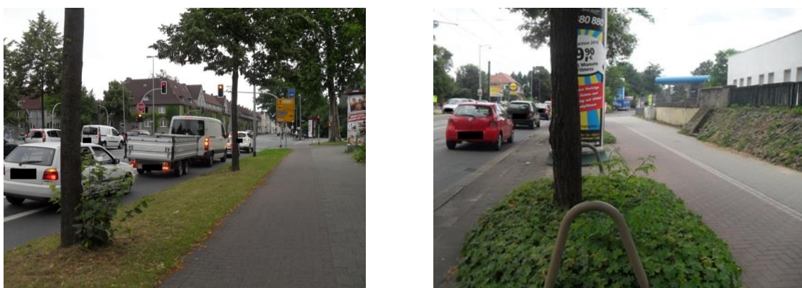
Figure 3.4. Examples of separated cycle lanes with potential line of sight obstruction in Germany. Source (Schreck & Seiniger, 2014).
