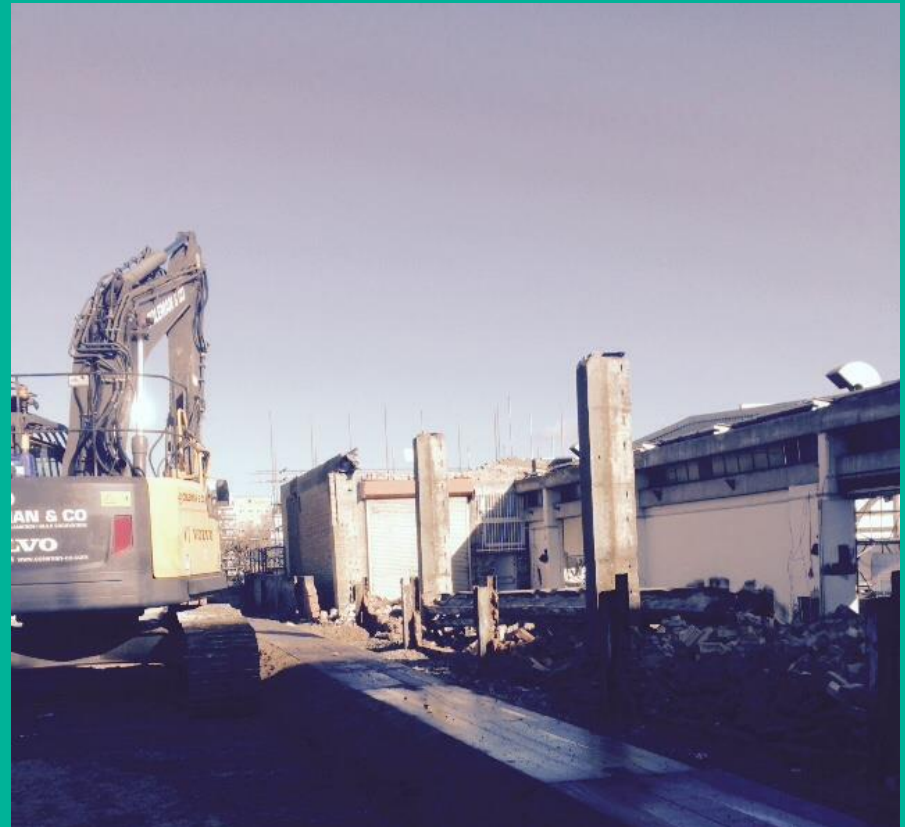
Demolition at CEMEX North
