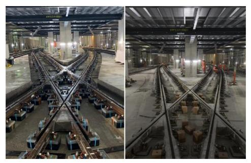
Fig. 3 & 4 Before (left) and after (right) concreting in the diamond cross over segment
