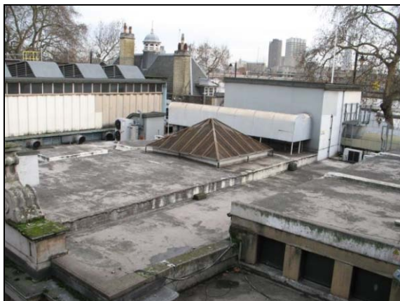
Embankment roof: before
