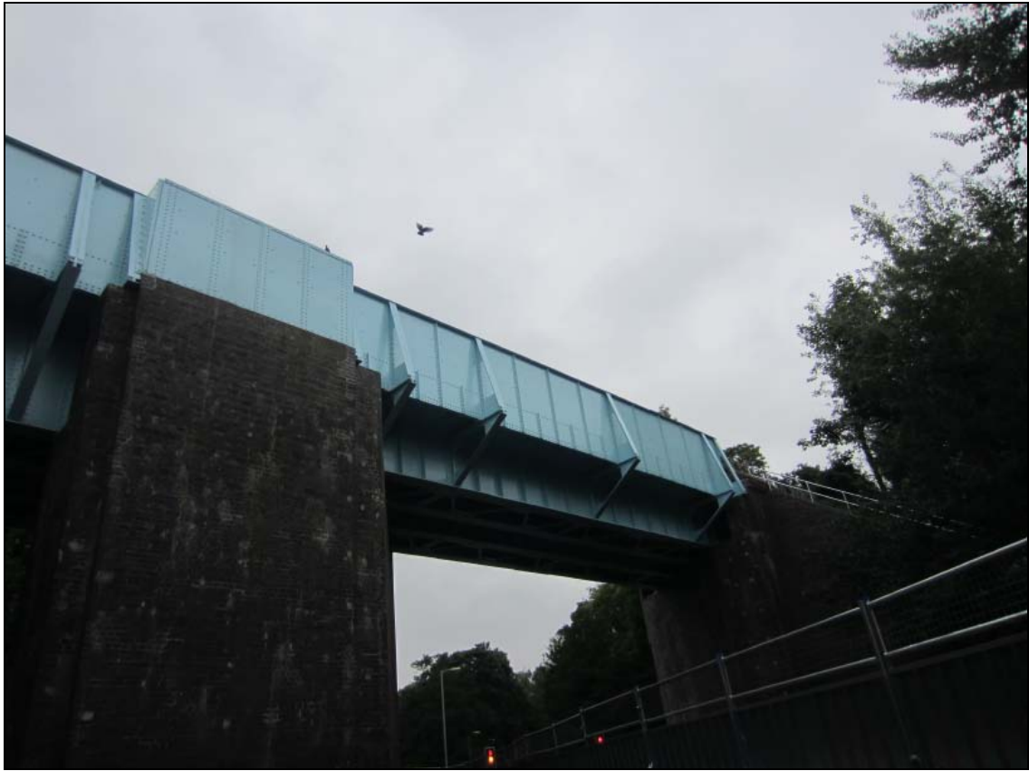
Newly painted bridge located between Watford and Croxley
