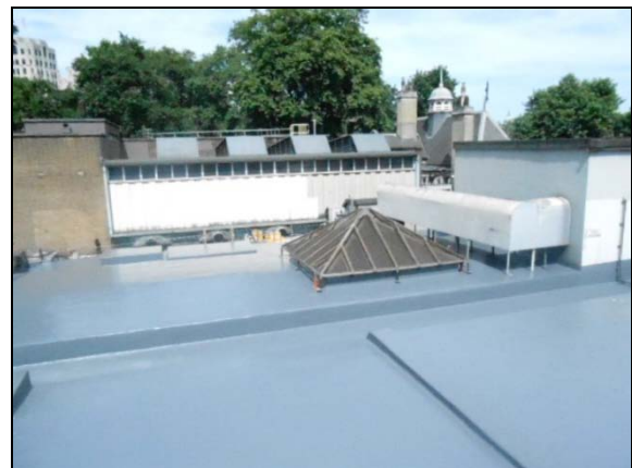
Embankment roof: after
