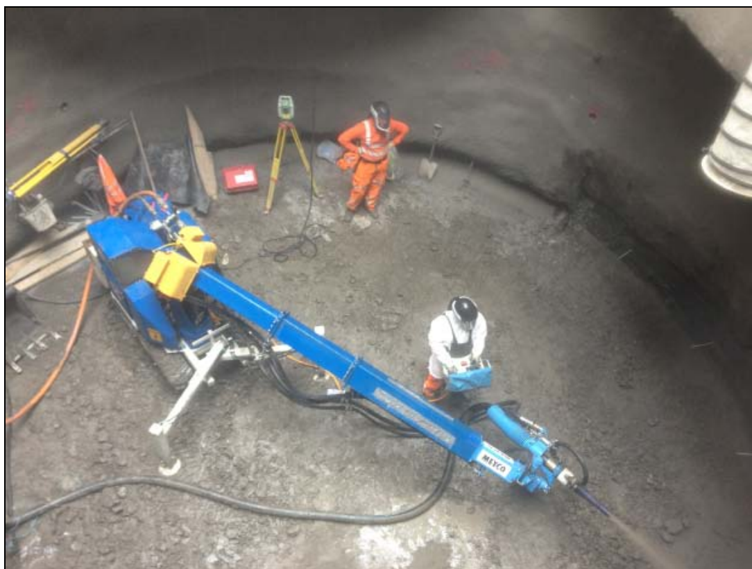
Bond Street concrete lining spray of shaft 1
