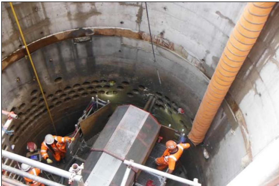
Bond Street shaft 5 with "tube-a-manchette" (TaM) drilling rig
