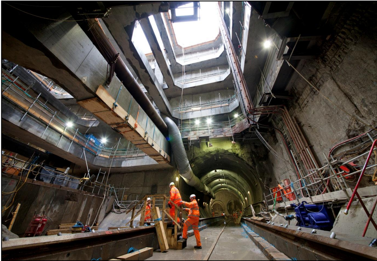
24 miles of train tunnels are due to be completed by spring 2015
