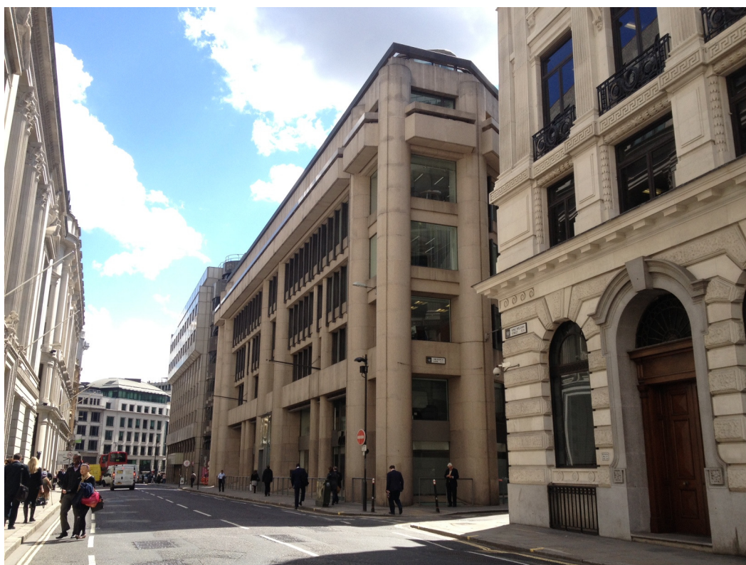
Plate 1: 10 King William Street from the north
