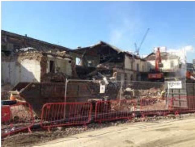
2) Banhams Demolition works
