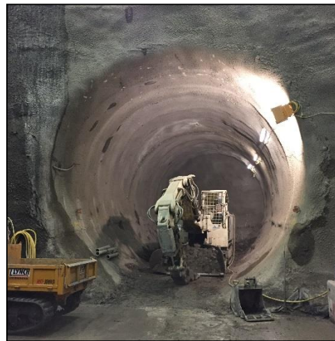
Completed Back Shunt Kennington Park
