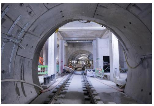
Image of the track intersecting the basement of the shaft
