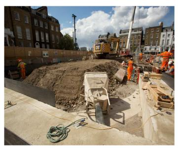
Concrete capping beam beneath acoustic enclosure foundations
