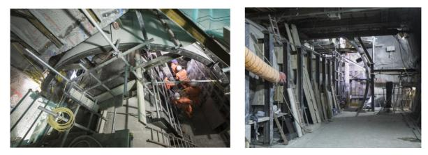
Above – image of the installation of the SGI rings and the tunnel support works.
