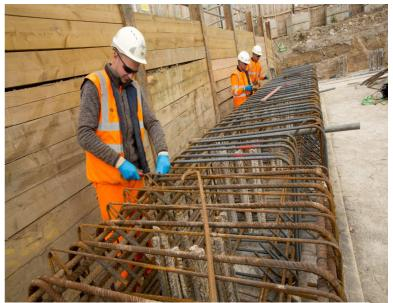
Preparation of the reinforcement cage for concreting
