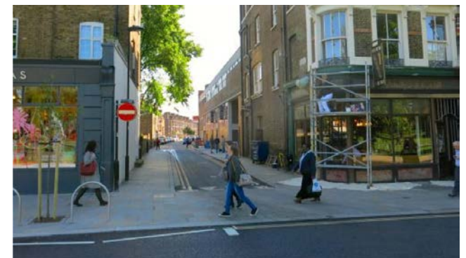
Continuous footway treatments in Lambeth
