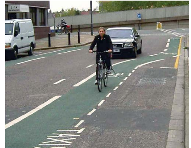
Advisory cycle lane marked around a taxi rank – lane would benefit from being wider or having a buffer to the marked rank
