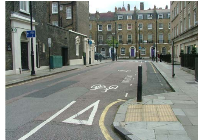
Footway build-out with contraflow cycle provision
