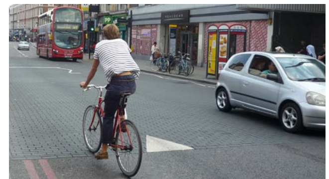
Imprint surfacing used for calming effect at pedestrian crossing at Kingsland High Street
