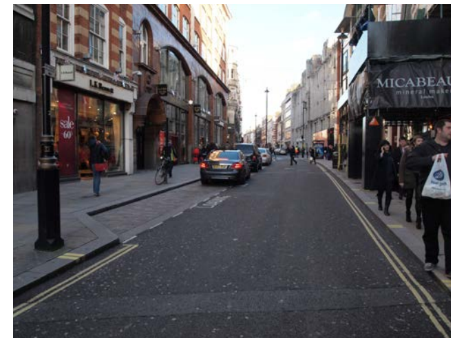
Fully inset loading bays to support retail premises – Long Acre, Covent Garden
