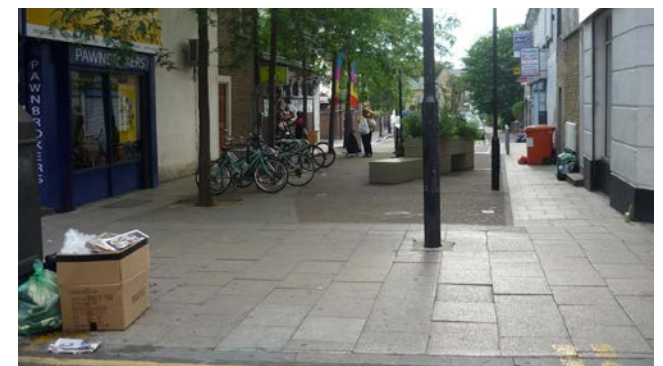
Continuous footway treatment in Hackney
