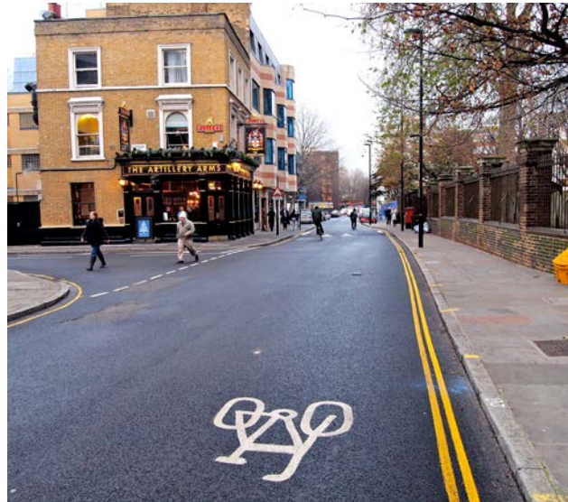
Minimal use of road markings – Bunhill Row
