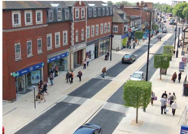
Narrowing through use of kerbed median strip, Hornchurch. Raised tables act as informal flush crossings.
