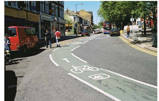
Cycle lane continued around bus stop cage
