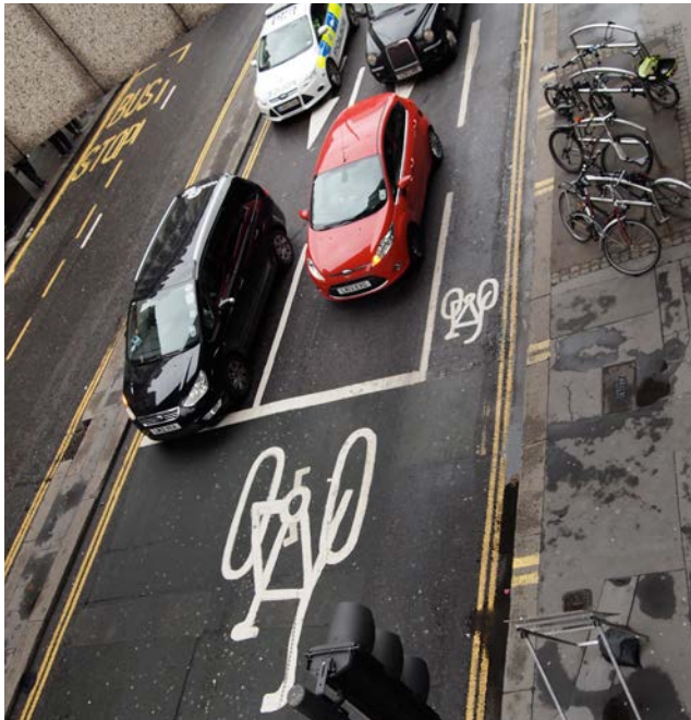
Traffic lanes narrowed to incorporate nearside feeder to an ASL – Aldersgate Street, City of London
