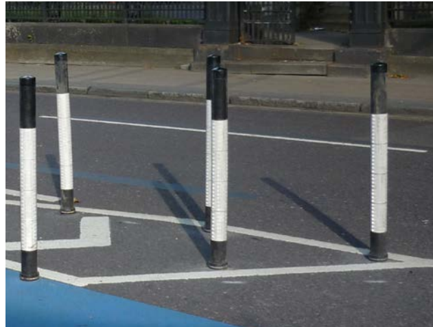
Flexible posts used for a temporary buffer to a cycle lane
