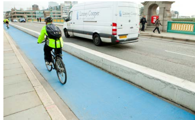
Kerbed separation, Southwark Bridge
