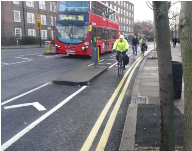
Cycle lane with buffer and intermittent island protection – Baylis Road, Lambeth
