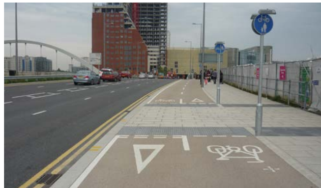
(Top) Raised delineator and ladder and tramline paving on a partially separated footway. (Bottom) Stop-start cycle facilities where partially shared provision briefly becomes a shared area
