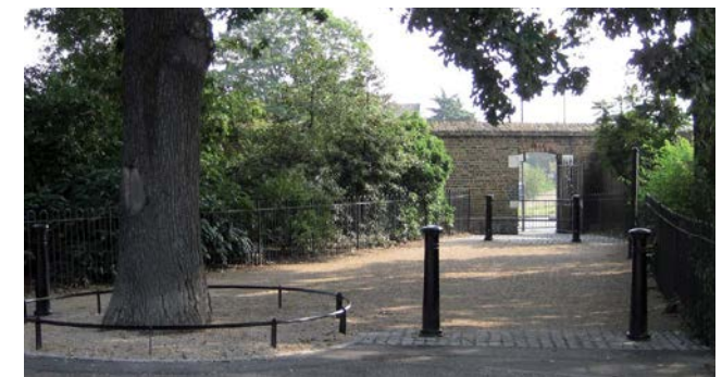
Improvements at Vanbrugh Gate, Greenwich Park. Before (top), barriers inhibit access by many types of user. After, barriers are more accessible, surface quality is improved, materials are better integrated with the setting and flush granite setts help to control cycle speeds ahead of the gate
