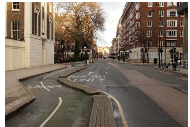
Track at Tavistock Street, Camden, forming a parallel carriageway and simplifying movement through a four-arm junction (but note the need for the left-turn ban).
