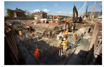
An overview from Wandsworth Road of the capping beam preparatory works
