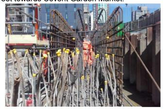
Steel cage reinforcement for capping beam installation
