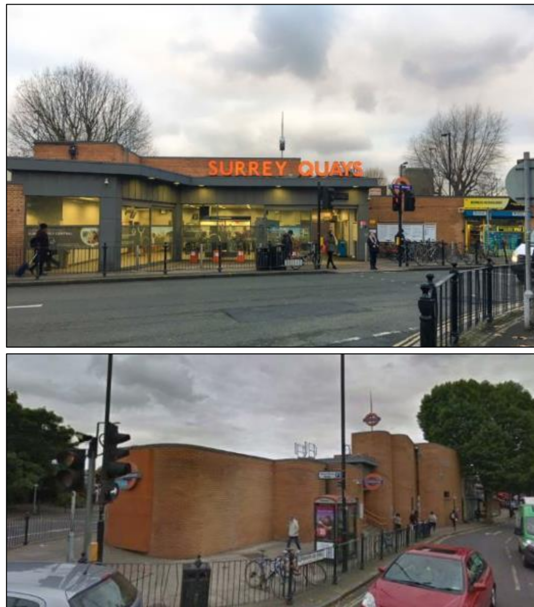
Figure 5-1 - Existing Station Building
