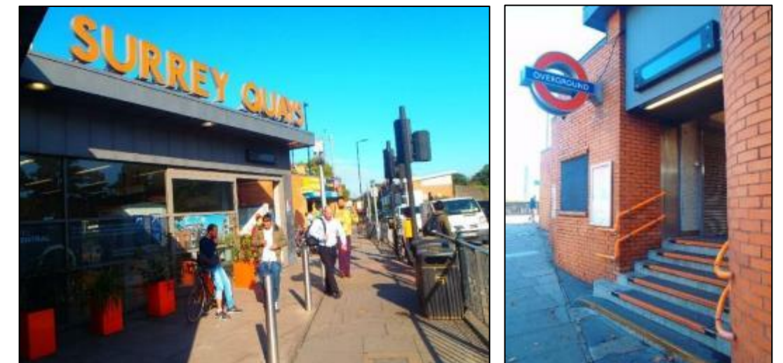
Figure 2-1 – Existing Station and Entrances on Lower Road and Rotherhithe Old Road Entrances
