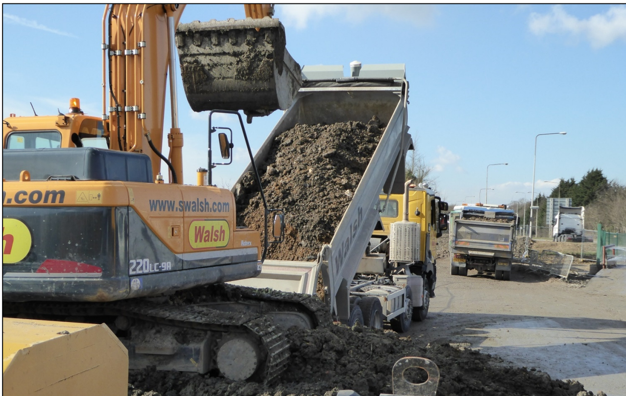
Figure 3-2 Paved tipping apron at entrance to landfill/remediation facility
