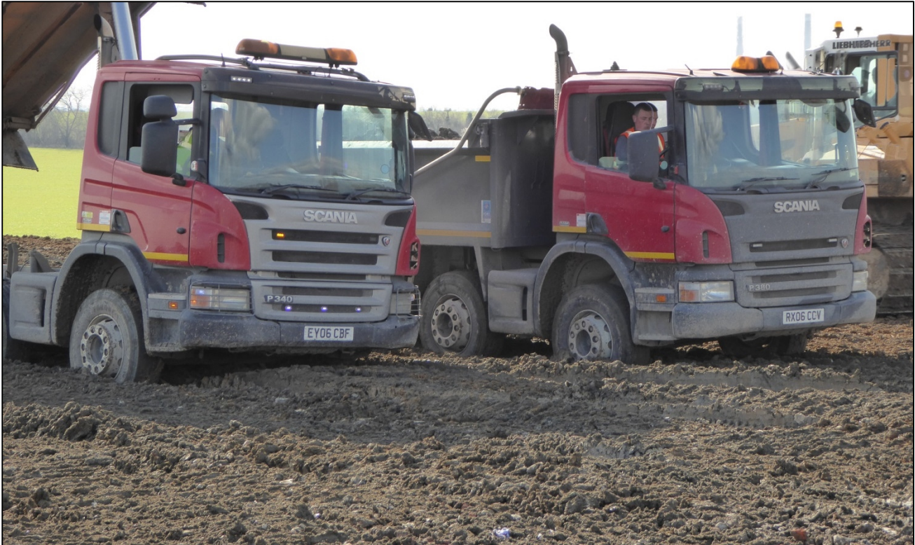
Figure 3-5 Ruts with the potential to cause damage to vehicles at tipping area
