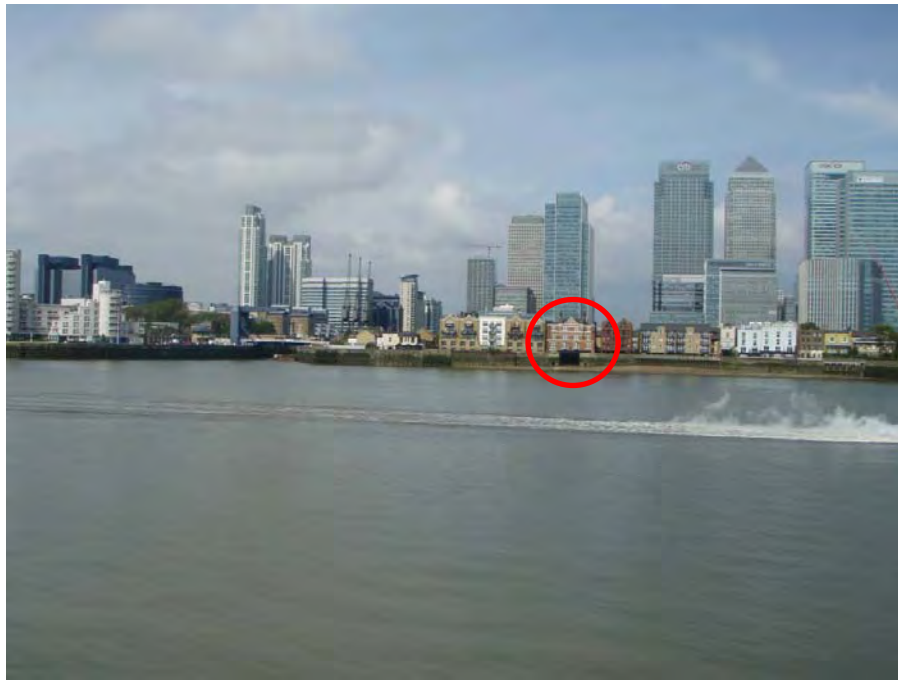
View of north bank (showing potential building to be acquired for demolition)
