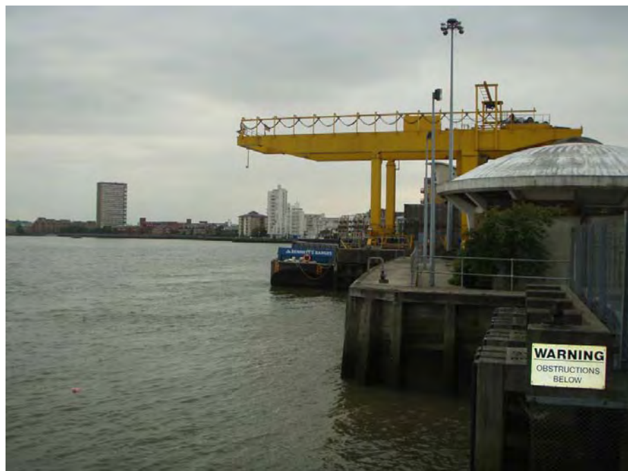
Northumberland Wharf recycling centre (working wharf) on north bank
