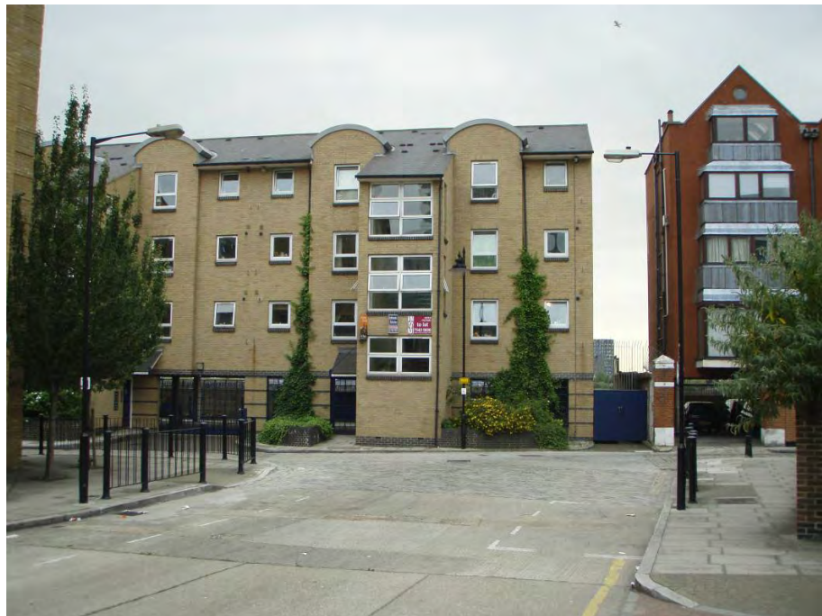
View on Coldharbour road (showing potential building to be acquired for demolition)
