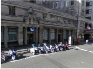
Clutter detracts from key building elements
