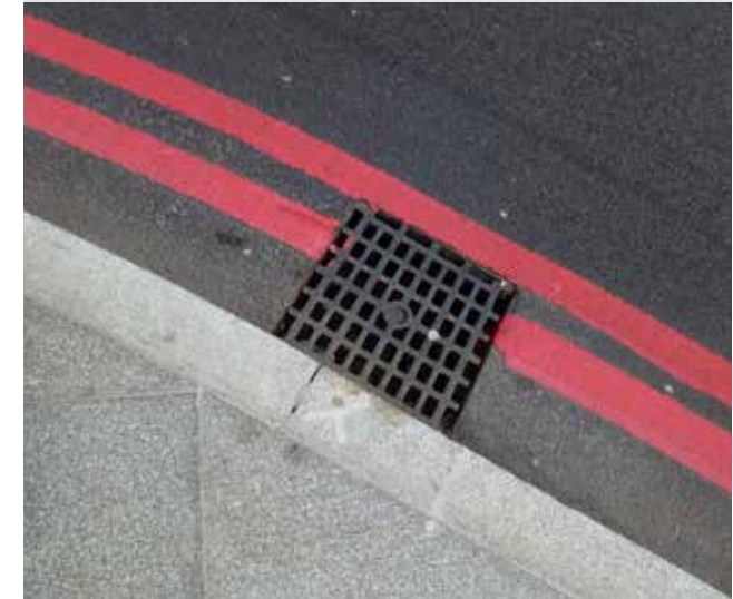
Figure 275: Cycle friendly grate on TLRN
