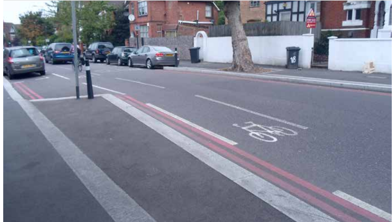
Figure 25: Ambleside Avenue was fully reconstructed
