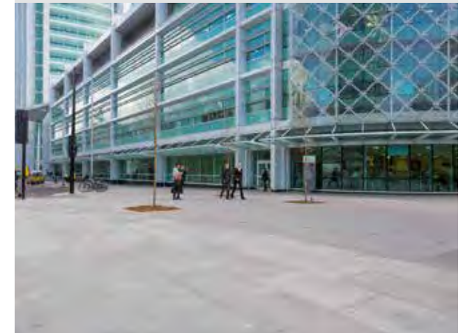
Figure 64: Euston Circus uses two shades of granite paving
