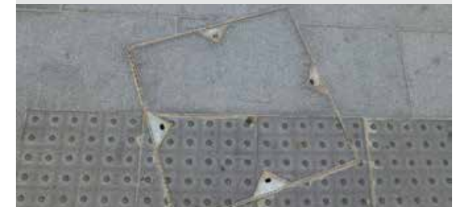
Figure 84: Granite tactile paving inset into an inspection cover
