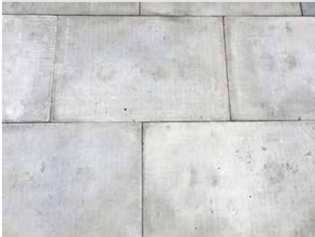
Figure 61: 900x600mm concrete slabs
