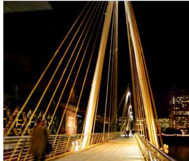
Figure 167: One of the Golden Jubilee footbridges
