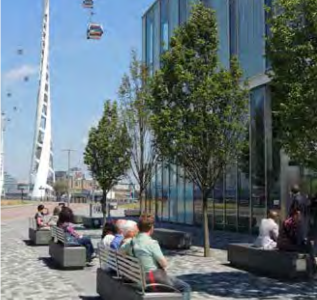
Figure 302: Emirates Air Line Greenwich Peninsula station where stone plinths are used as a security measure and a seating feature
