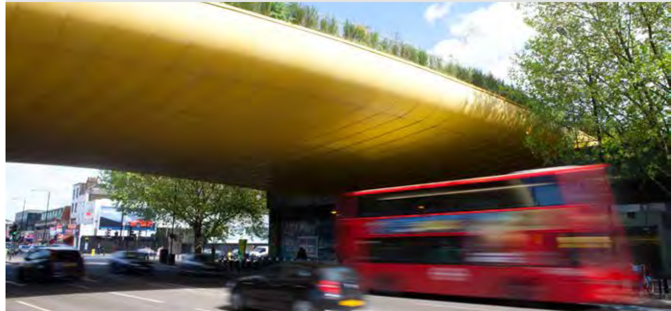
Figure 172: Bridge creating a friendly urban environment under its structure
