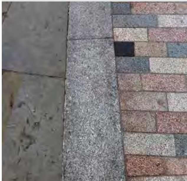
Figure 75: Yorkstone transitioning to granite setts with a flush granite kerb acting as a border
