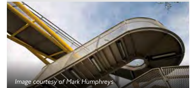
Figure 169: Necessary structural elements can be designed to be beautiful elements in their own right
