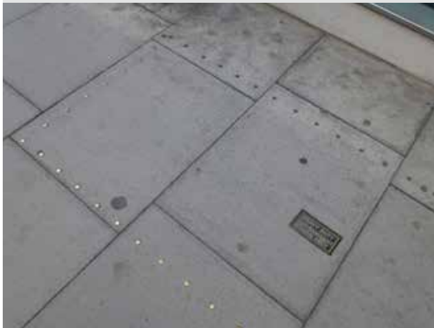
Figure 92: A smoke vent demarcated with studs and an inscribed metal plate
