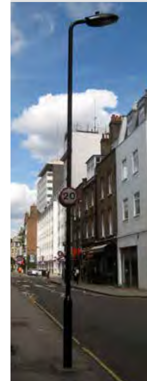
Figure 285: Example of a stepped tubular column
