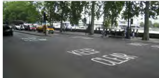
Figure 106: Victoria Embankment: 'Keep clear' markings have been used instead of a yellow box
