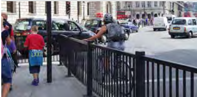
Figure 254: Guardrailing often restricts free movement by non motorised users
