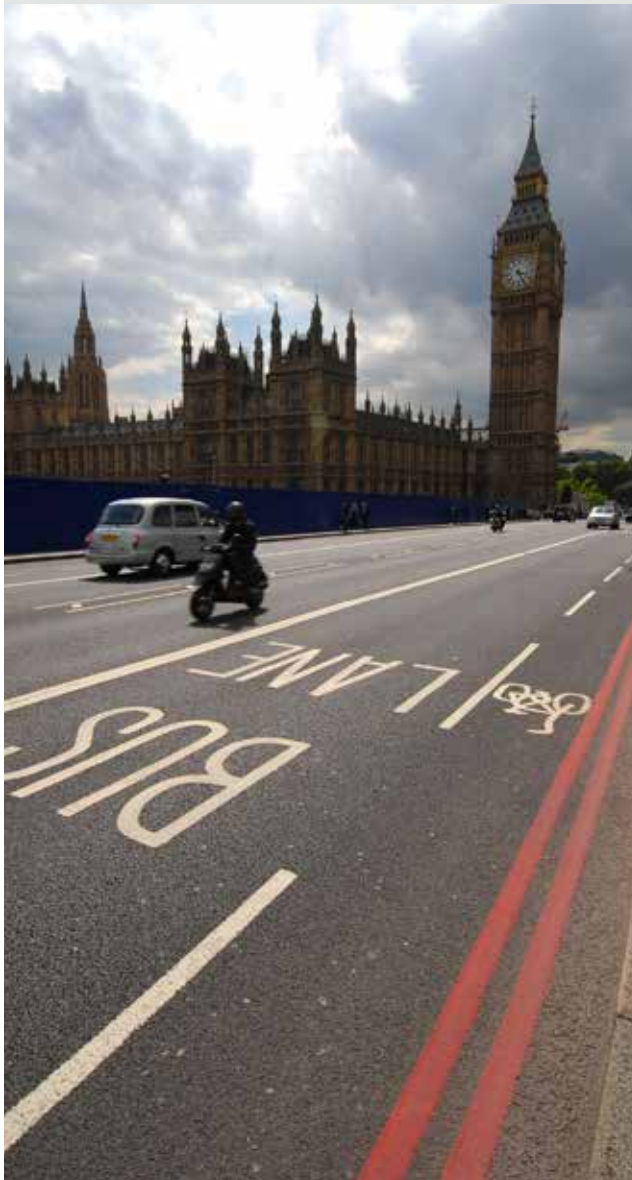
Figure 114: Bus lane and advisory cycle lane on Westminster Bridge
