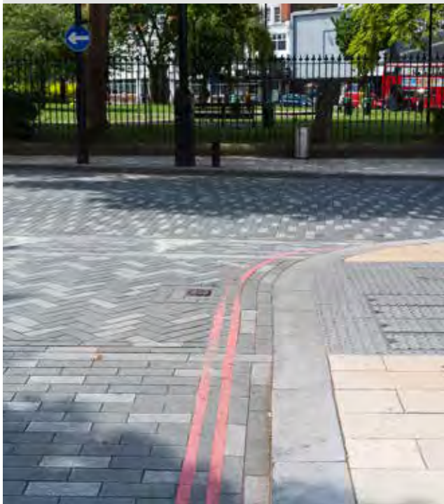
Figure 153: A side road entry treatment at Windrush Square, Brixton
