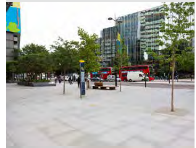
Figure 78: A private development transitions subtly to the TLRN through use of similar materials and coordination with the streetscape
