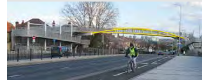
Figure 168: The bright colouring of this bridge acts as a beacon in the streetscape
