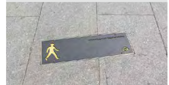
Figure 240: Legible London temporary foundation cover plate
