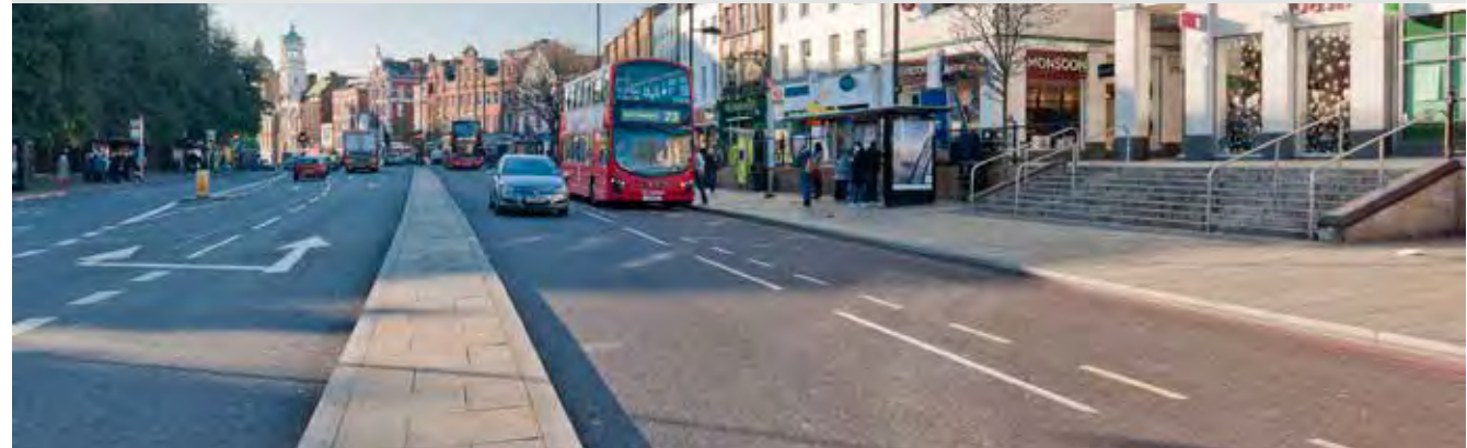
Figure 20: A series of interventions at Angel town centre has led to a more user friendly street with increased space allowance for pedestrian movement and a negligible impact on vehicle capacity
