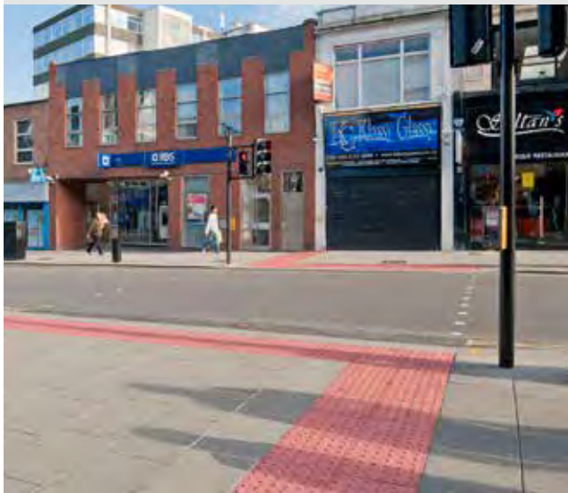
Figure 138: A Ped-X crossing on Harrow Station Road with no pedestrian countdown timer
