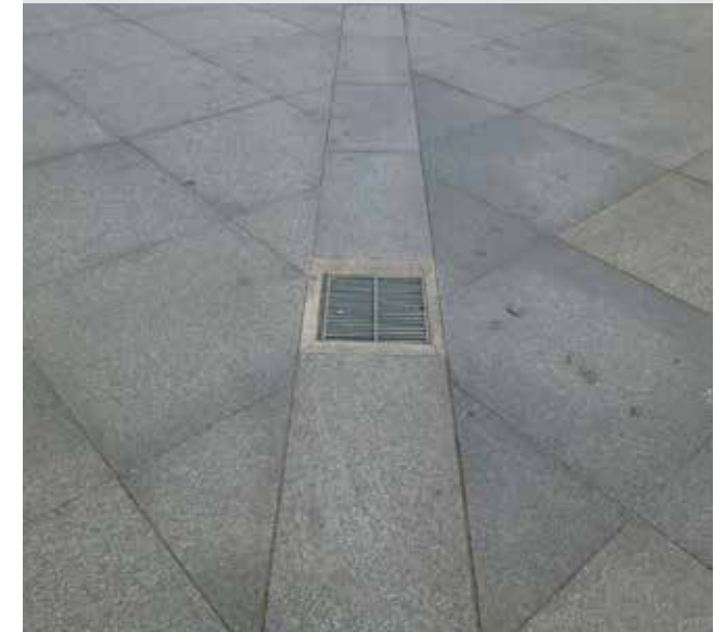
Figure 276: Channel and pedestrian friendly gully
