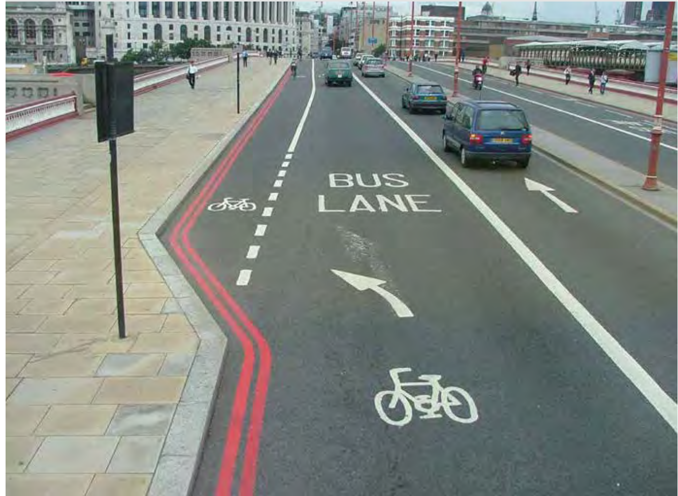
Figure 110: Blackfriars bridge mandatory cycle lane
