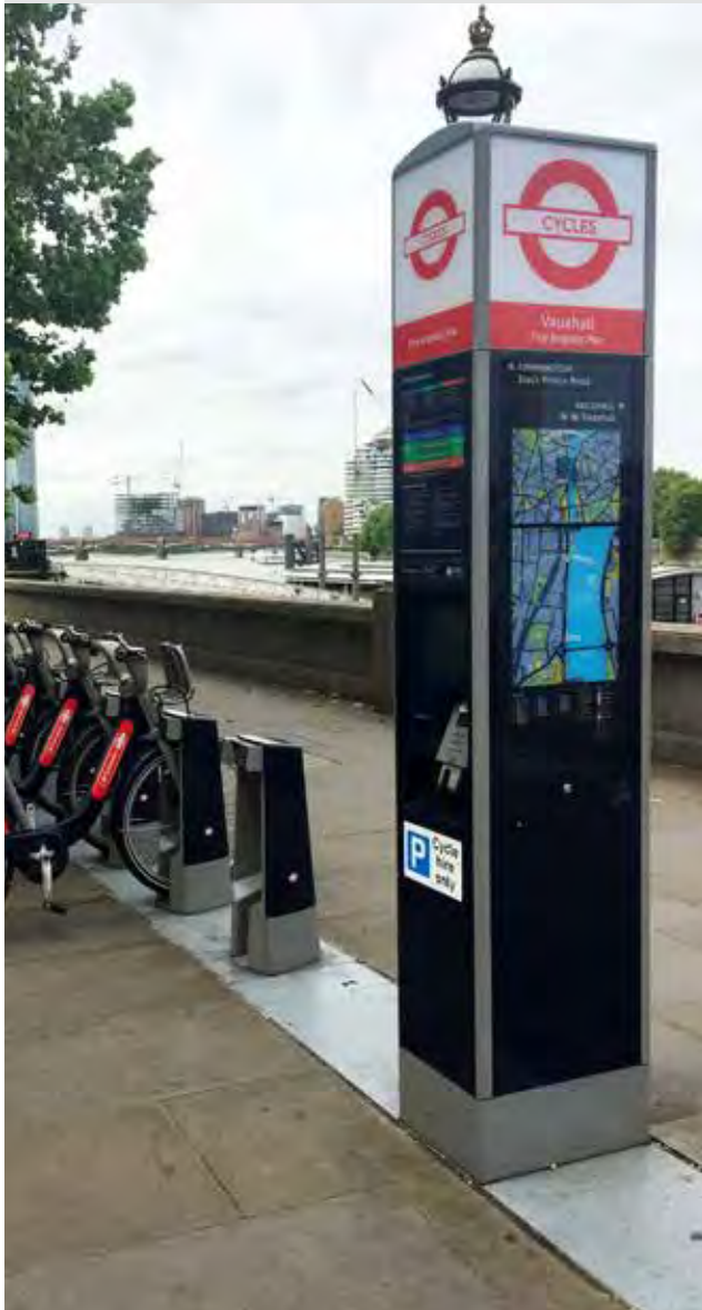
Figure 218: A cycle hire docking station on Albert Embankment
