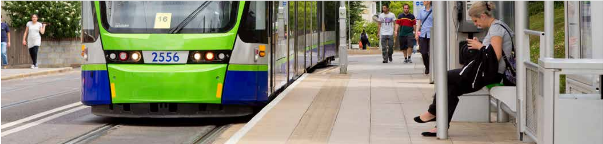
Figure 135: Lozenge paving at a tram stop
