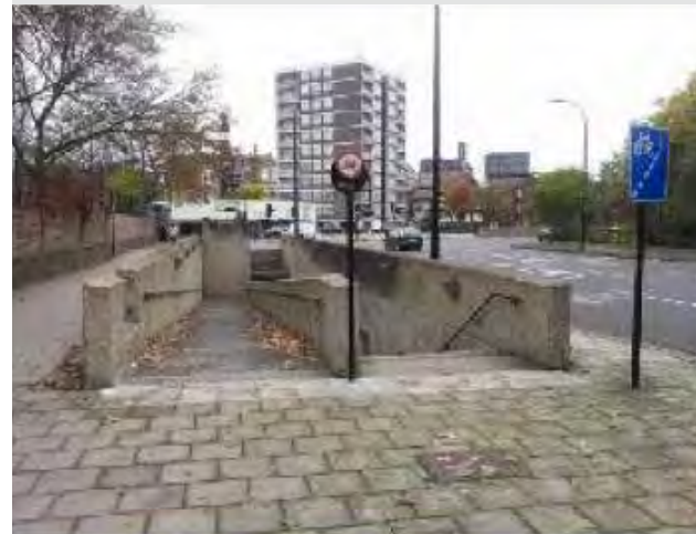
Figure 163: Bricklayers Arms roundabout subway closure in Southwark, before and after
