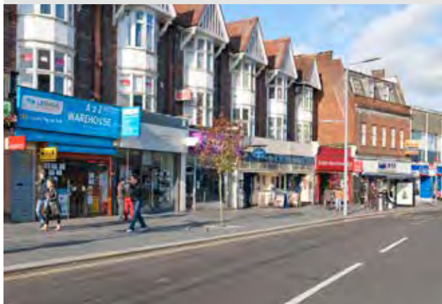
Figure 211: Advertising boards correctly placed on Station Road in Harrow
