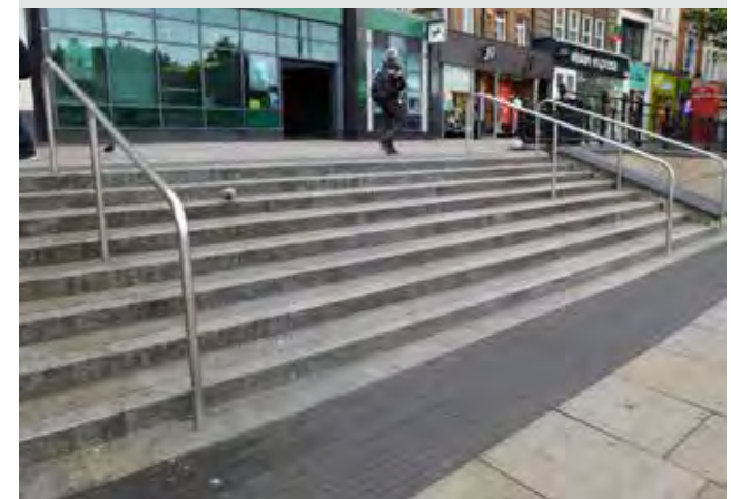
Figure 133: Corduroy paving used at stairs to indicate a level change
