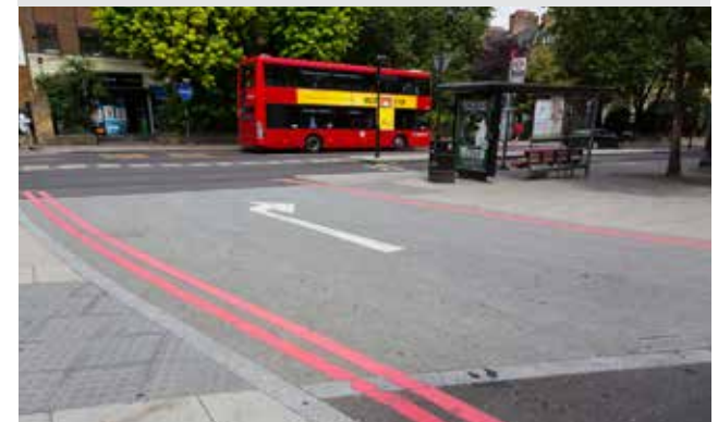
Figure 102: Granite setts on a raised table at Goswell Triangle
