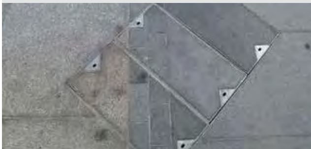
Figure 85: Paving pattern inset into an inspection cover
