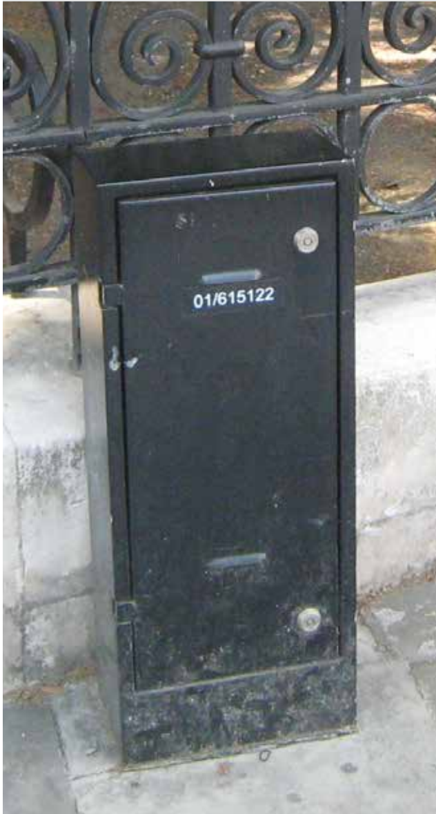
Figure 259: Pillars should be placed away from pedestrian desire lines
