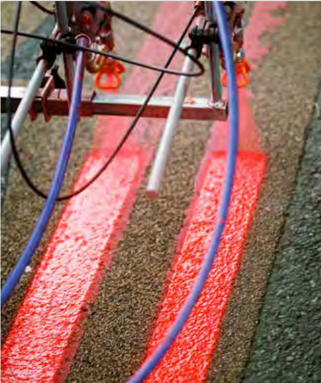
Figure 108: Renewed red line markings
