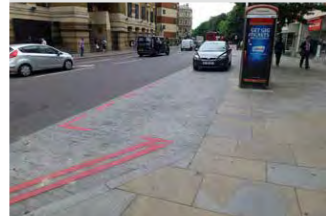
Figure 175: A parking bay paved in granite setts extends the footway when not in use
