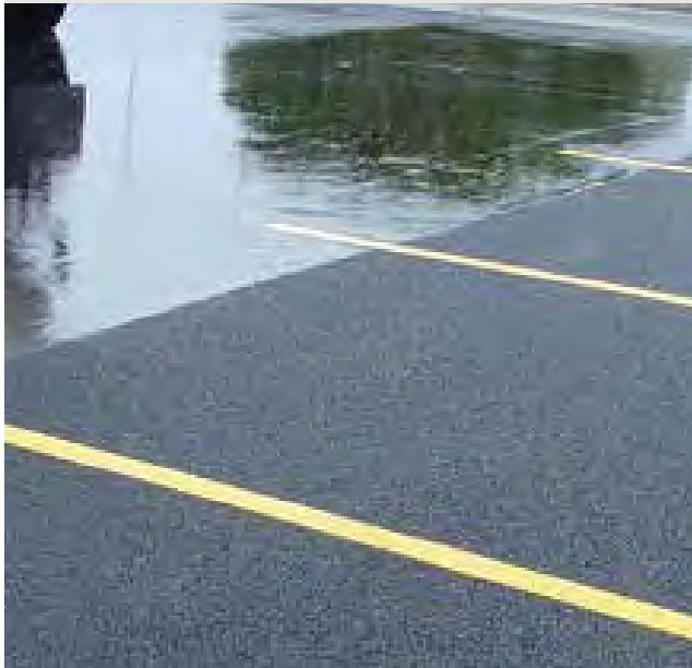
Figure 37: Permeable asphalt allows water to infiltrate
