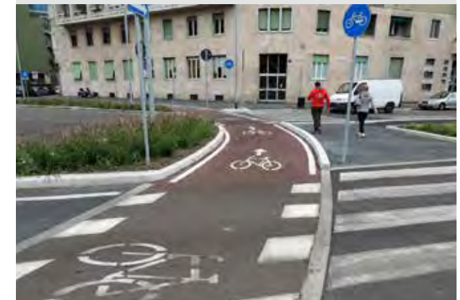
Figure 147: A zebra crossing with a parallel cycle crossing in Milan
