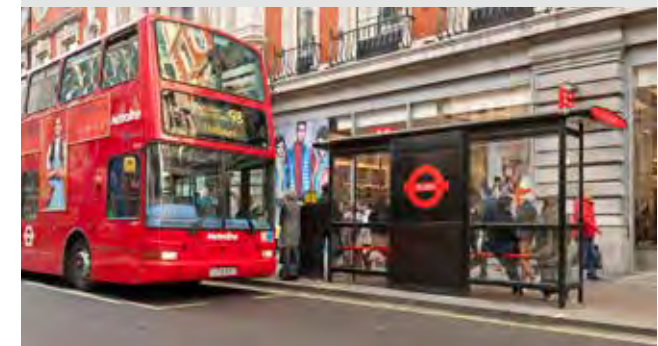
Figure 195: A bus stop on Oxford Street with the shelter orientated with the back to the kerb
