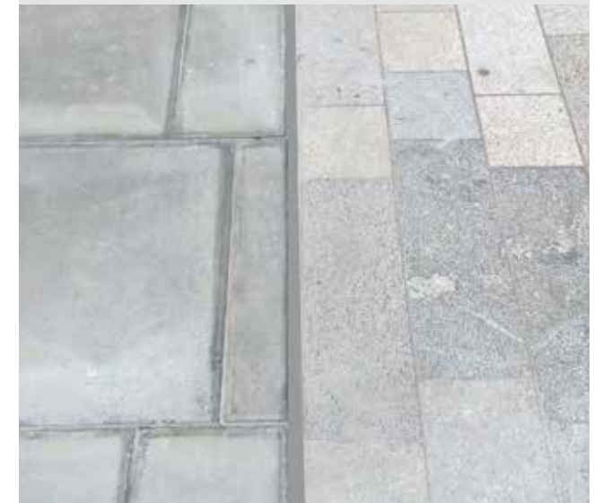
Figure 76: 900x600mm concrete slabs transitioning to granite
