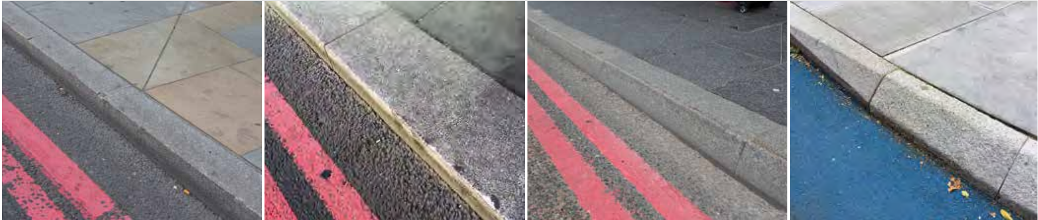
Figure 95: A selection of kerbs on the TLRN
