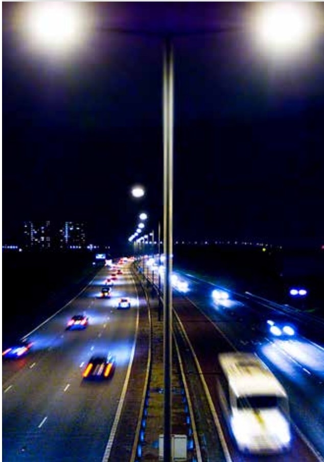
Figure 35: CMS is being installed on street lights across the network
