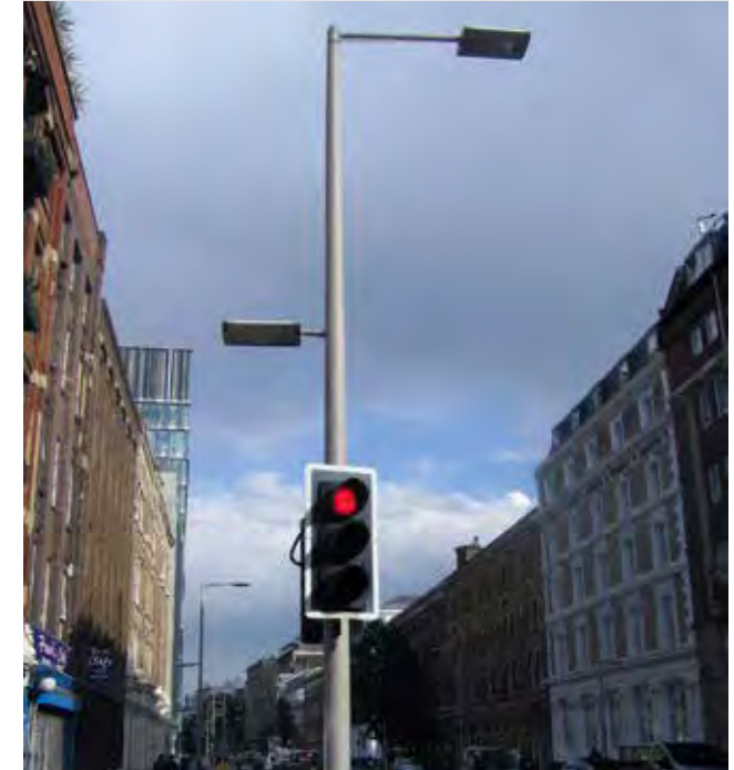
Figure 290: Combined lighting column and signal head
