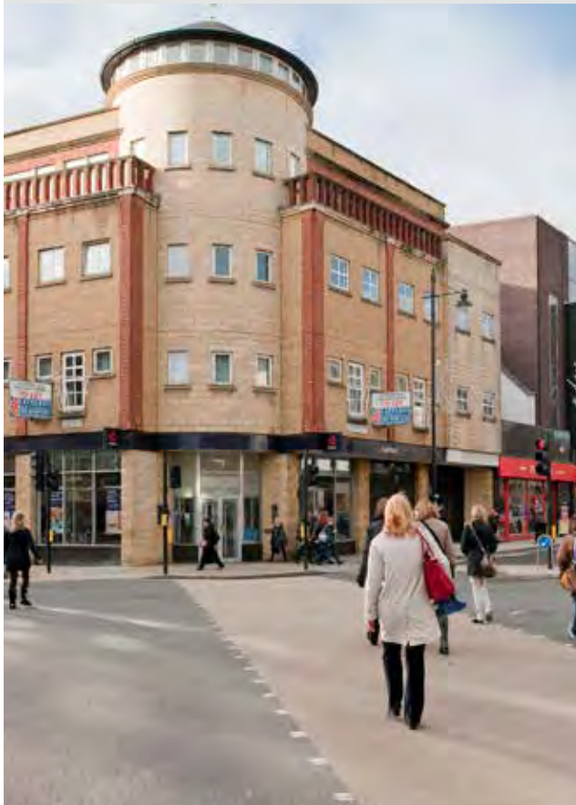
Figure 145: Diagonal crossing in Wimbledon
