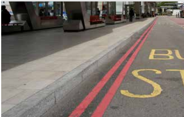
Figure 301: Bus interchange with a 140mm kerb upstand
