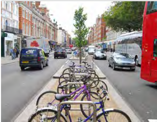
Figure 119: The central median on Kensington High Street utilised for cycle parking and tree planting
