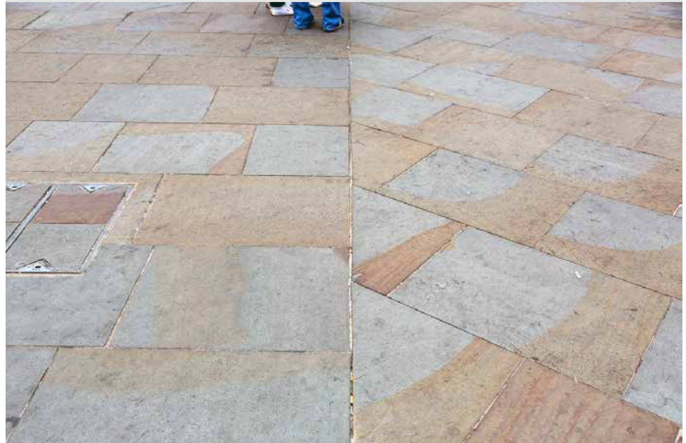
Figure 69: Careful attention should be given to the treatment and appropriate cutting at locations where surface materials of different types or alignments join. The footway on the left side of the cut line shown in this image has taken precedence, as the primary road of the two
