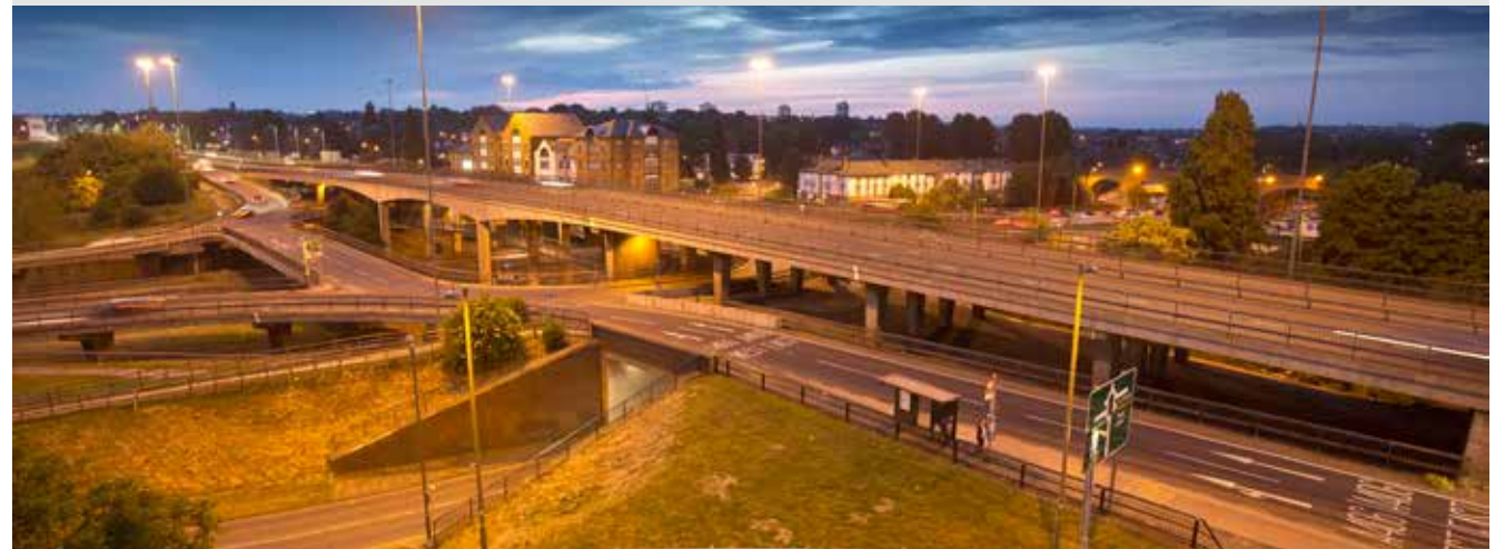
Figure 287: CMS is used to control lighting levels throughout the hours of darkness
