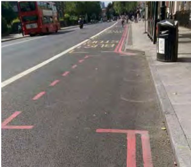
Figure 190: A bus boarder used to raise the kerb height to 140mm
