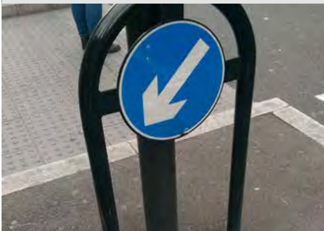
Figure 212: A 'keep-left' hoop bollard illuminated by carriageway lighting
