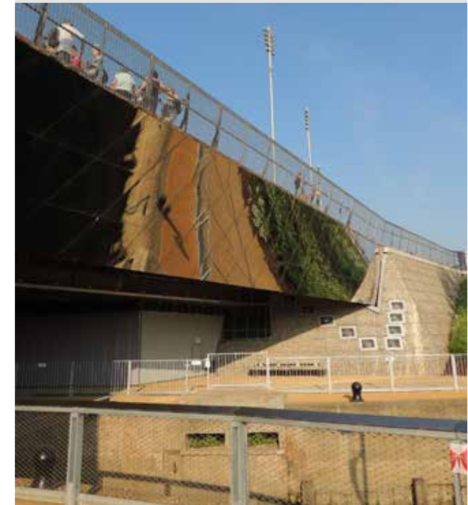
Figure 160: A footbridge in Queen Elizabeth Olympic Park in Stratford, London
